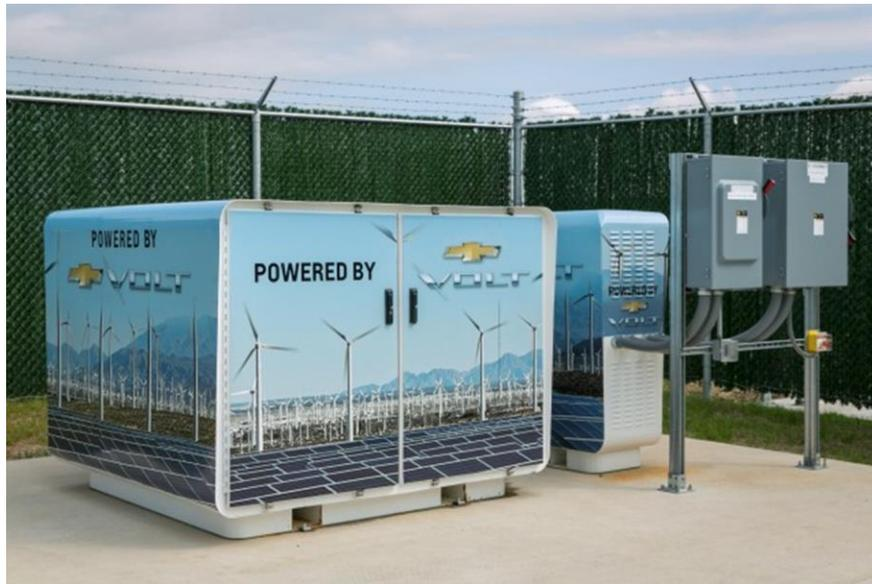
**Figure 14 Energy Storage Facility Using Chevrolet Volt Batteries at GM Facility in Milford, Michigan**
