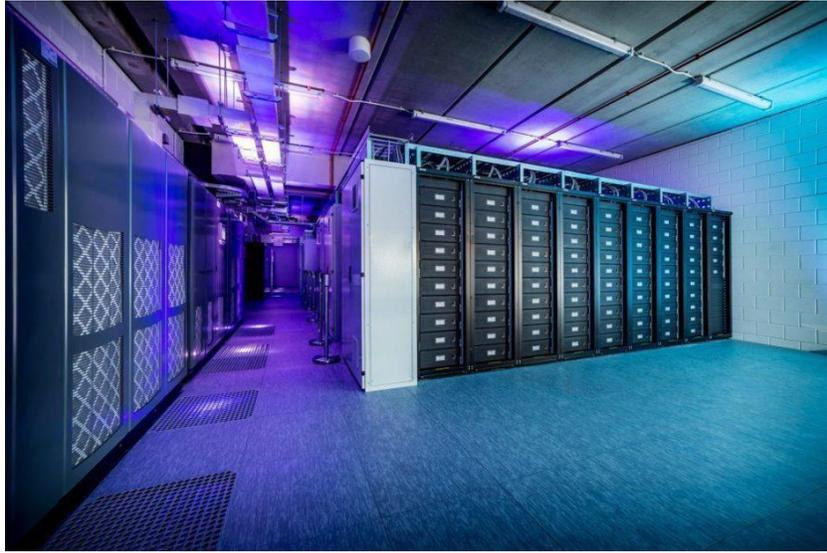
**Figure 73 The Mobility House – EV Batteries Used for Energy Storage in Nissan-Eaton Partnership<sup>410</sup>**
